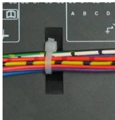
With Cable And Tie In Place
